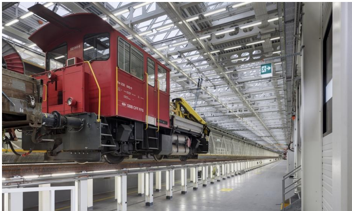
Production facilities for railway operations
