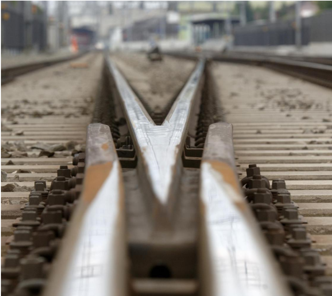
(1) switch blades / switch points (2) stock rail (3) locking (4) switch rod / tie bar (5) machine (6) crossing / frog (7) guard rail
